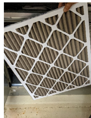
Figure 2. Example eSpin pleated filter (after use)
