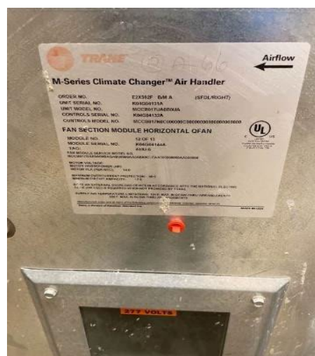
Figure 2-11. Air Handler Name Plate
