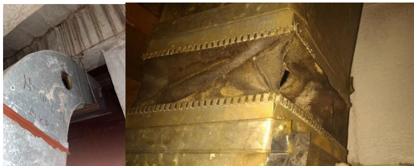
Figure 2-14. Duct Hole and Hole in Canvas Connector
