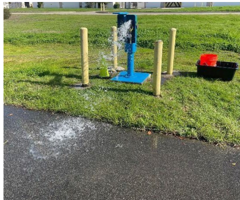
Figure ES-5. A Leak Simulated at the Sampling Station During Phase-I Testing.
