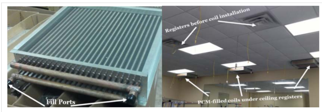
Figure 4. PCM-Filled Ceiling Coils
