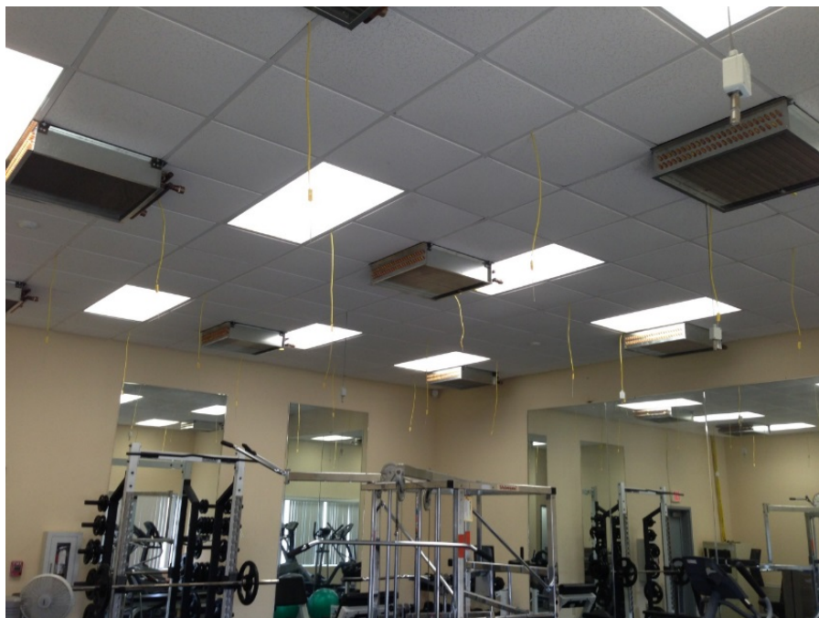
Figure 20: Exercise room complete ceiling coil installation
